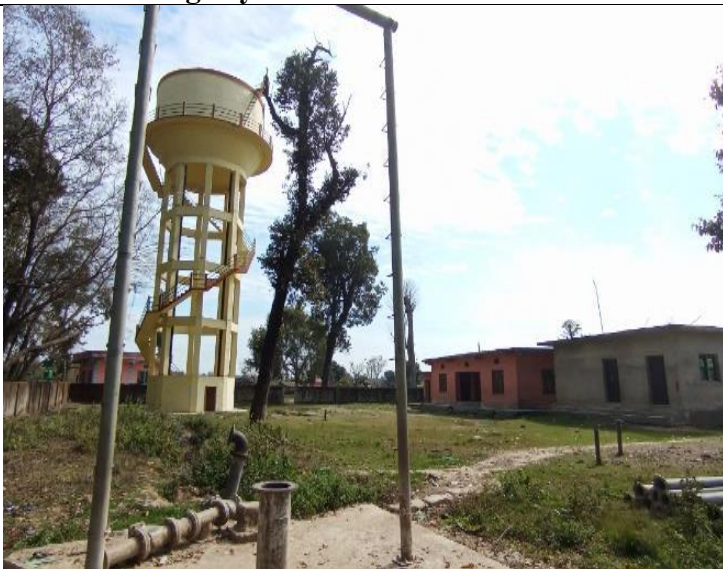
3. Existing structure at the Ranikunda WSS sub-project, OHT premises
